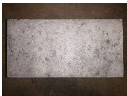
Fig. 10 Condition of top surface
