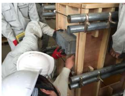
(2) Install of BOSS mold
