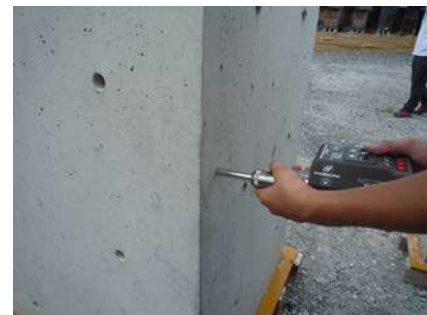
Fig.6 Rebound number test
