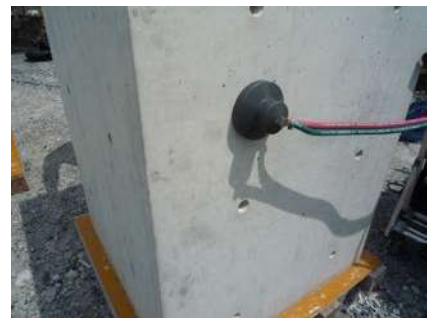
Fig. 5 Air permeability test
