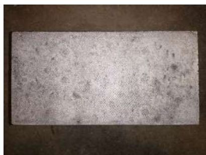
Fig. 10 Condition of top surface
