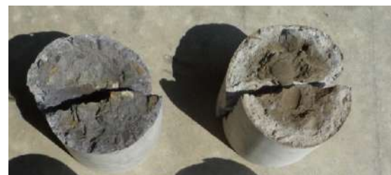
Discolored boundary by chloride ions
