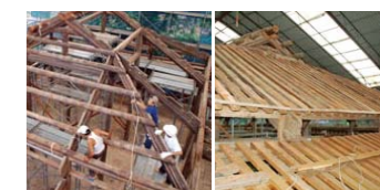
2008 隆徳殿の母屋取付 2008 隆徳殿の垂木取付
