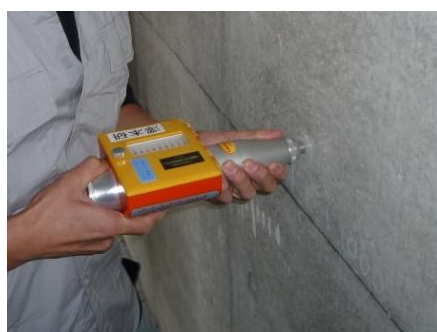
Fig. 1 Rebound number test
