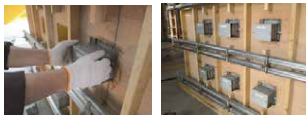
Fig.3 Installation of Cube BOSS mold
