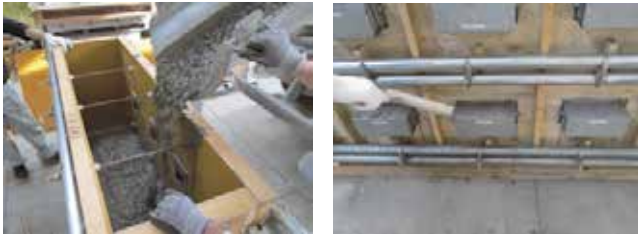
Fig.4 Placing of concrete to wall specimen
