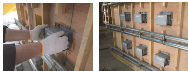
Fig.3 Installation of Cube BOSS mold
