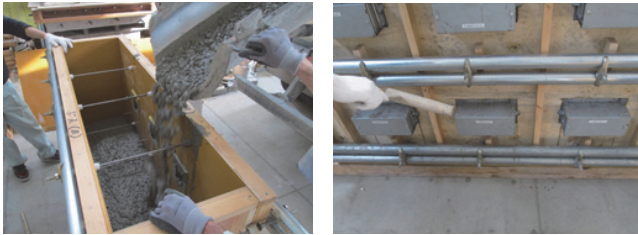
Fig.4 Placing of concrete to wall specimen
