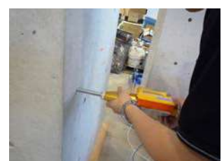
Fig. 6 Rebound number test
