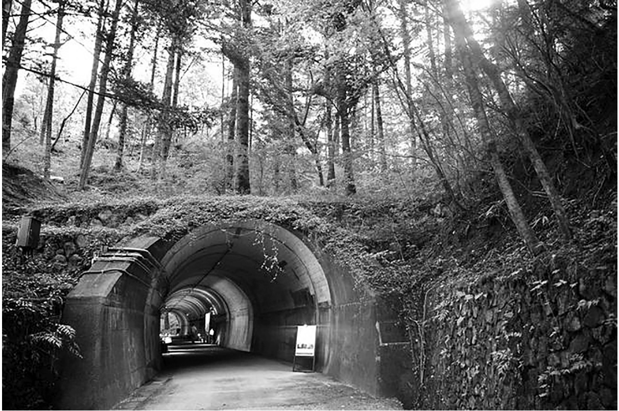
The entrance to the Aoba tunnel is surrounded by trees. (Takuya Tanabe)
